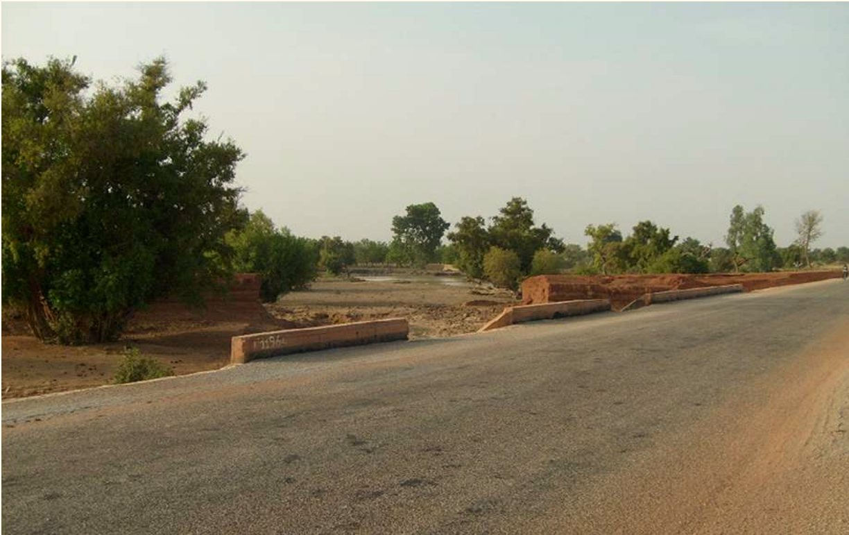
Figure 15. The newly paved road RN22.
