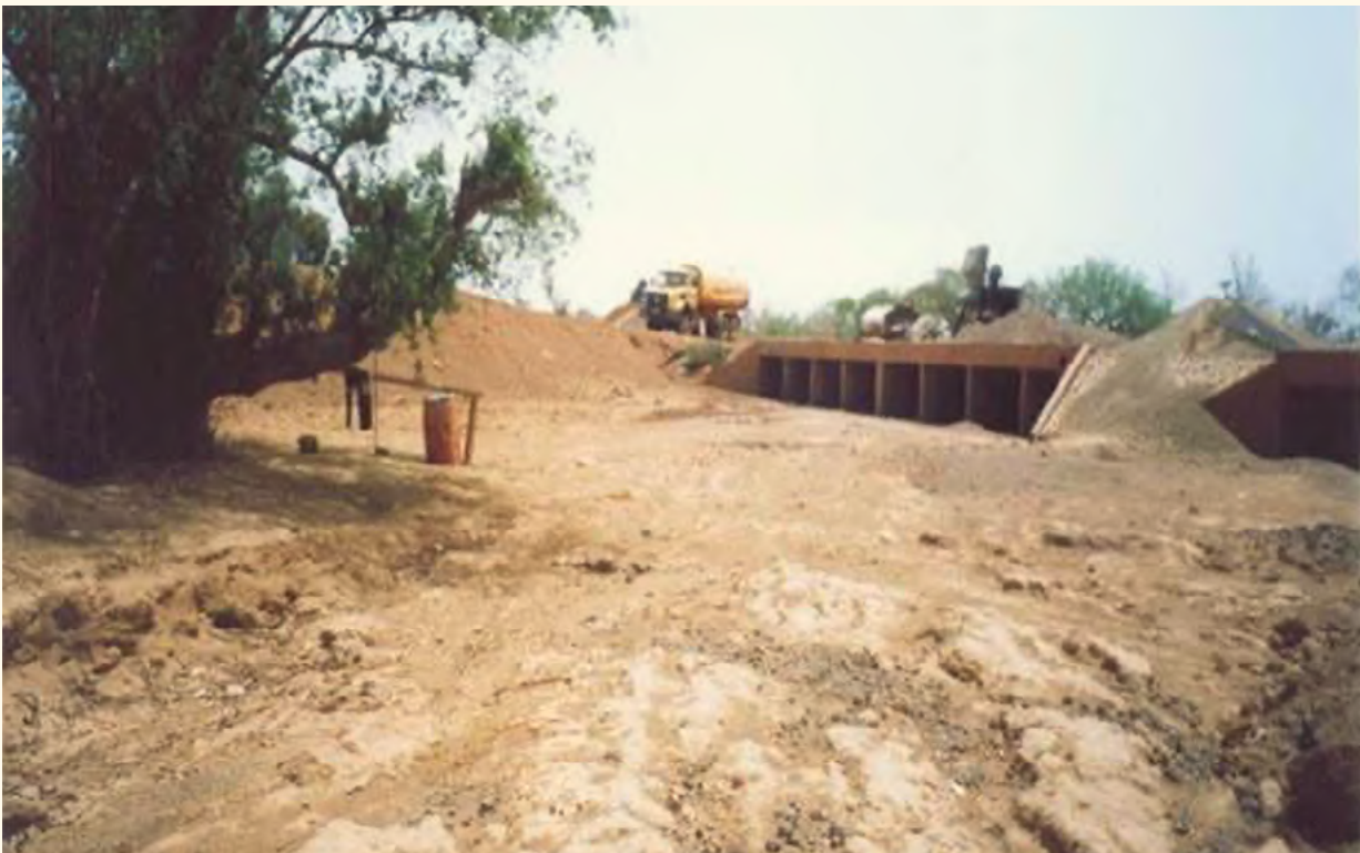
Figure 13. The dry riverbed downstream of the dam.
