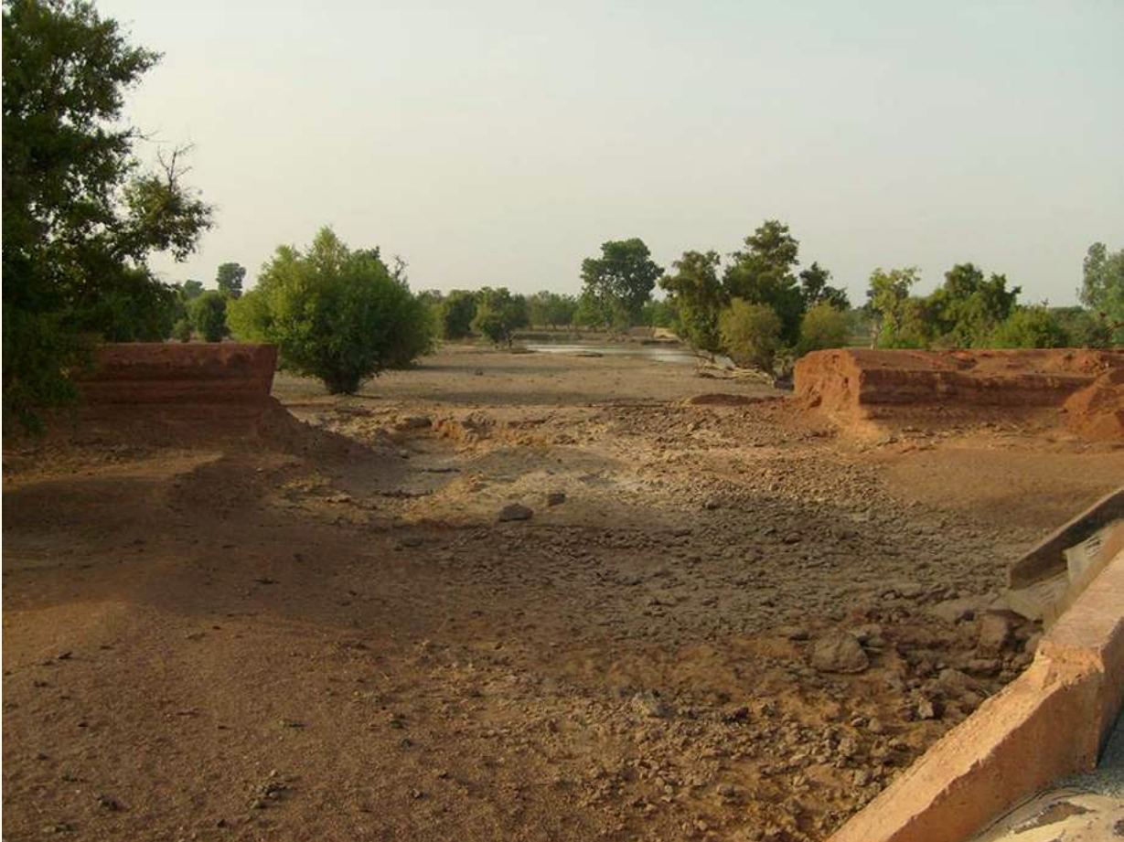
Figure 14. Opening the dam in the riverbed, October 2007.
