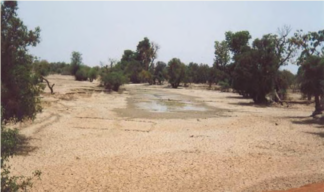
Figure 12. The dry riverbed upstream of the dam.
