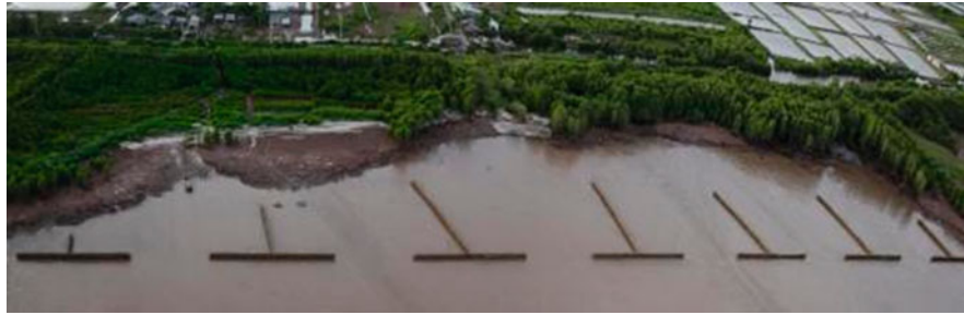
Fig. 9 Restoration of eroded floodplains using T-shaped bamboo fences in Bạc Liêu Province (Mekong Delta, Vietnam). The long-shore elements close the eroded gap in the mangrove forest by connecting the remaining headlands. They reduce incoming wave energy while the cross-shore constructions reduce the long-shore currents. The gaps between the long-shore elements allow for faster sediment input during flood tides and enhance drainage during ebb tides. The latter will accelerate the consolidation process of the sediment deposited inside the fenced area (Photo: Cong Ly and GE Wind 2013)
