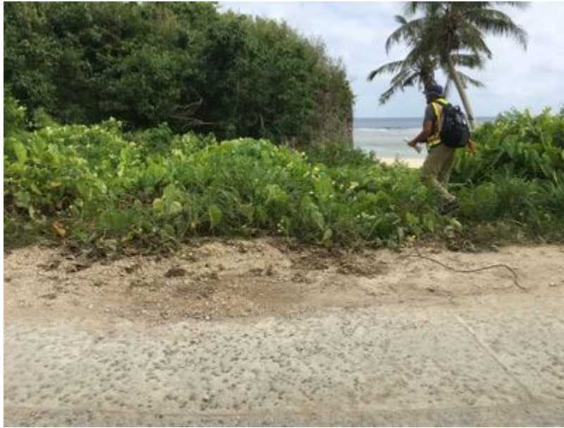
Additional Photo Caption: intended flow path middle left (pile of dirt). Current flow path on right.
