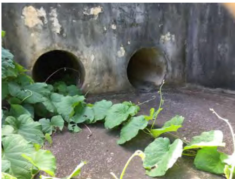
Additional Photo Caption: Headwall on downstream end
