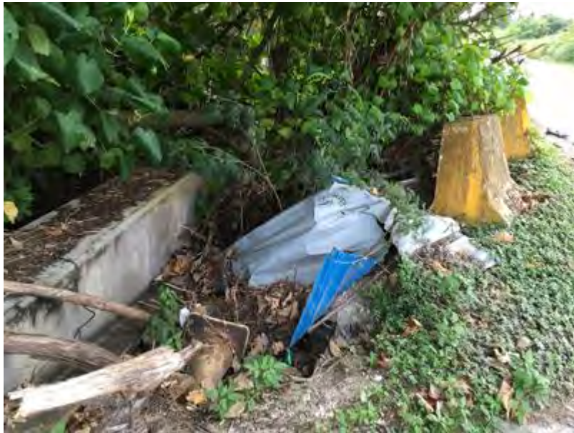
Additional Photo Caption: Trash near headwall of culvert (left)
